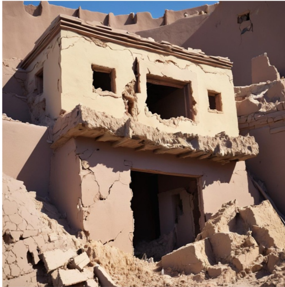
House built on sand
